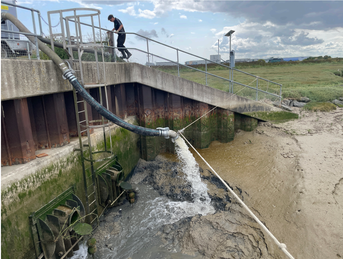
Fig. 20: Hicks 2023. Desilting. Sluice, Great Stour, Reach 9, Sandwich Town Tidal Defence.
