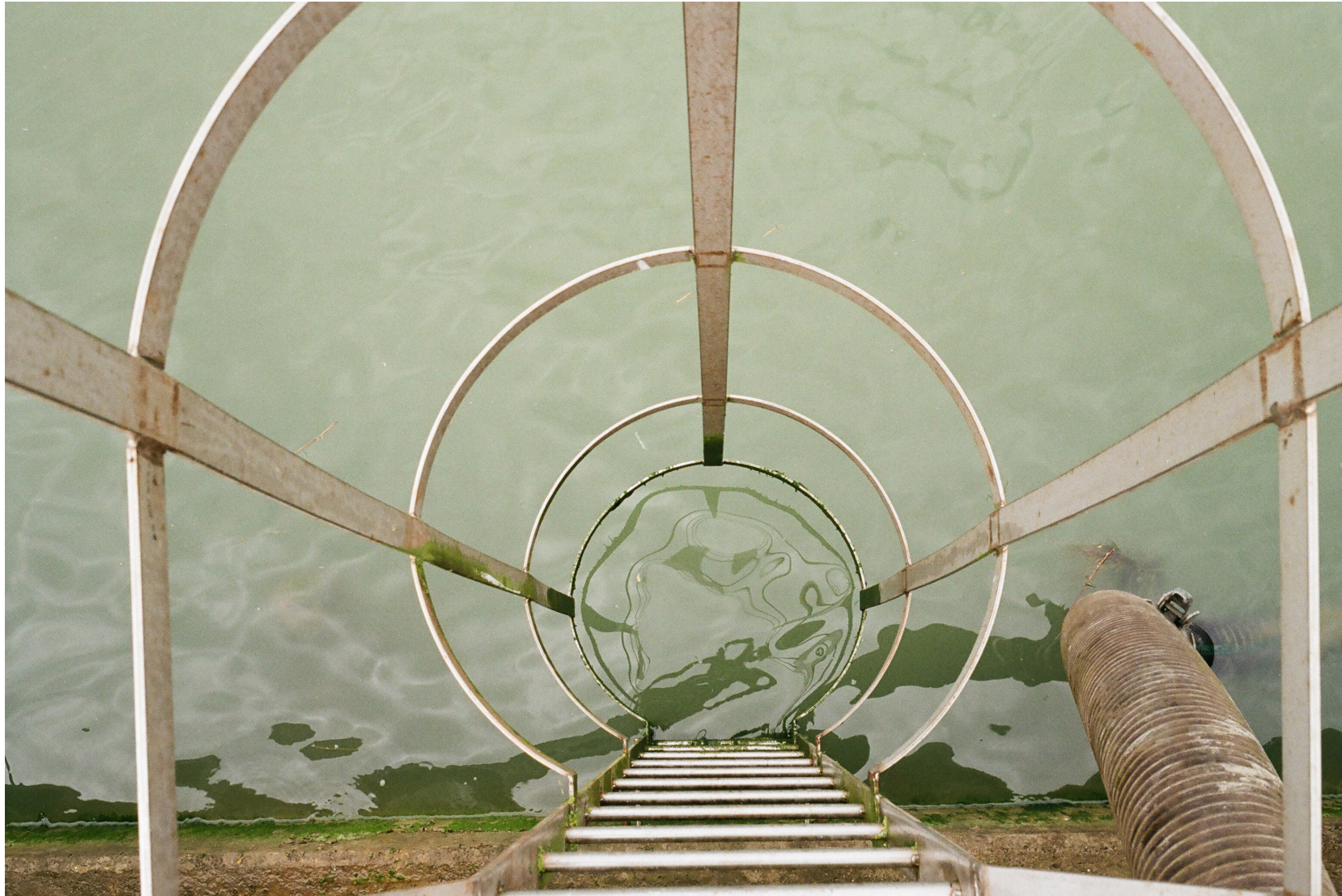
Fig. 18: Hicks 2023. Restricted access. Sluice, Great Stour, Reach 9, Sandwich Town Tidal Defence.
